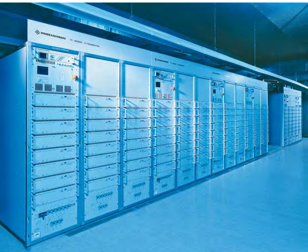
FIG 1 The transmitters in the Munich Olympic Tower cover the Munich/Southern Bavaria area.
